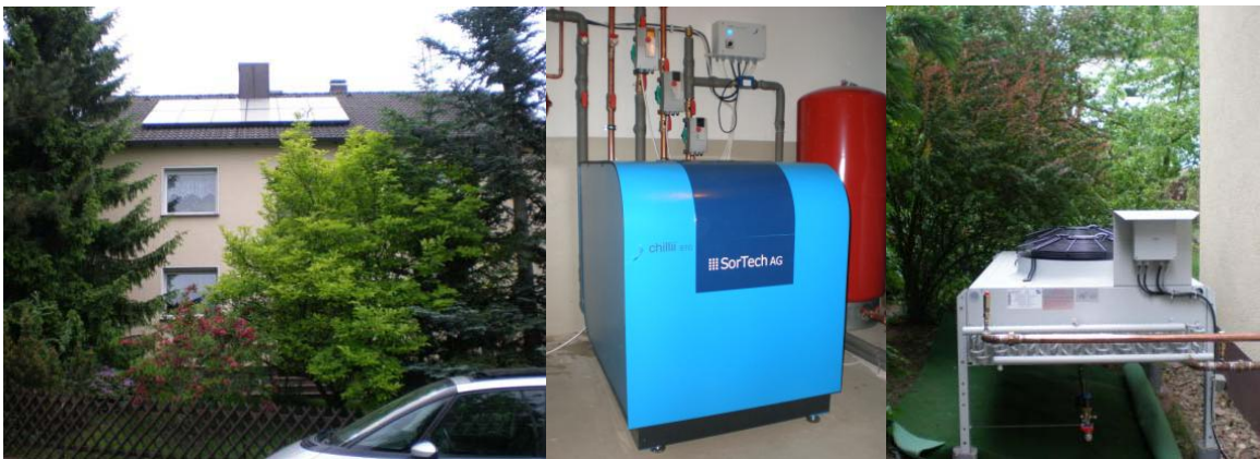
Fig. 5. Flat plate collectors on the roof of the two-family-house as well as the chillii ® STC8 adsorption chiller and the dry re-cooler (sources: SolarNext).
