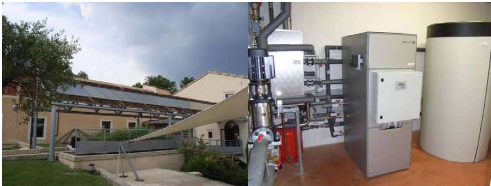
Figure 3: Building integrated flat plate collectors of the Haribo Museum in Uzés, France and suninverse 10 in the technical room (sources: Sonnenklima)
