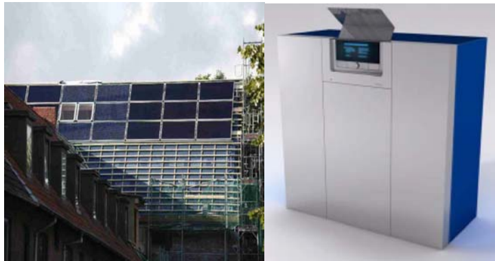
Figure 2: Roof-integrated flat plate collectors of the solar cooling system Buddenhagen and absorber LB 15 (sources: Schüco)
